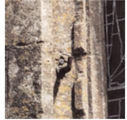
1.1.2. The holes left by the withdrawal of the pintles. These are sometimes left open, but have usually been filled with mortar or cement. Where modern colour-matched mortars have been used by conservators the repairs can be very difficult to identify.
