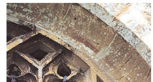
3.2. Where the mouldings of the window jamb contained flourishing lichen communities the edge of the frame may have either scraped these away where the board chafed when it was opened (or installed), or have changed the microclimate so that the original colonies have died off, ceased to develop, or been replaced with different species, leaving a vertical line on the jamb coinciding with the edge of the frame or shutter
