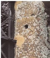
1.1.5. The replacement of a whole jamb stone may be an indication of the former presence of a pintel where there is clear evidence for two or more of the others elsewhere in the window.
