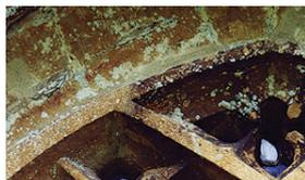
3.3. Occasionally an original sill stone may exhibit a line of natural weathering erosion - either continuous or as a series of pits - coinciding with the line of the lattice or the shutters when closed. This has presumably formed as rainwater dripped off the bottom edge of the frame.
